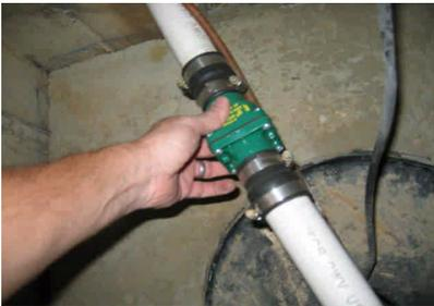
A check-valve is installed on the sump pump's discharge pipe. Good.
