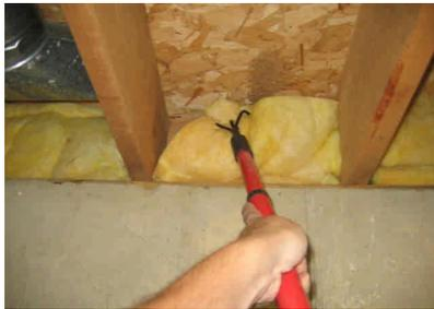
The floor joists are made of dimensional wood lumber - 2x10s.
