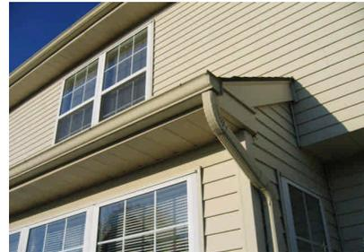
The vinyl siding appears functional. No major damage or deterioration was apparent. Recommend monitoring during a rain storm to see how the siding repels water. Be sure that the places where siding meets a different material is sealed or water-tight.
